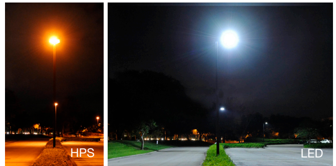
The images above compare LED fixtures versus High Pressure Sodium (HPS).
