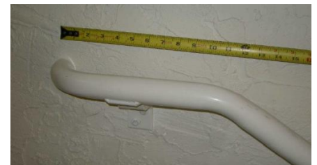
Example of compliant handrail at top riser
